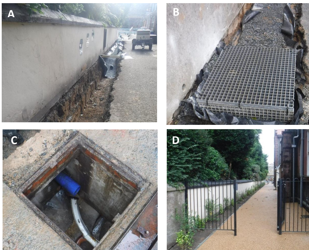
Figure 3: Installation stages of the vegetated swale channel; (A)Excavated trench with 160mm perforated pipe laid to a fall towards (B) the basket which housed inlet, outlet and high level overflow connections to (C) the existing chamber. (D) Shows the completed swale with initial
