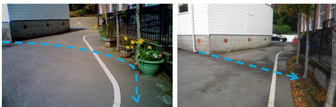
Figure 4: Removing old tarmac from around trees (left) has allowed for bioretention where rainwater from the white music building runs to naturally and is now used by the trees (right).
