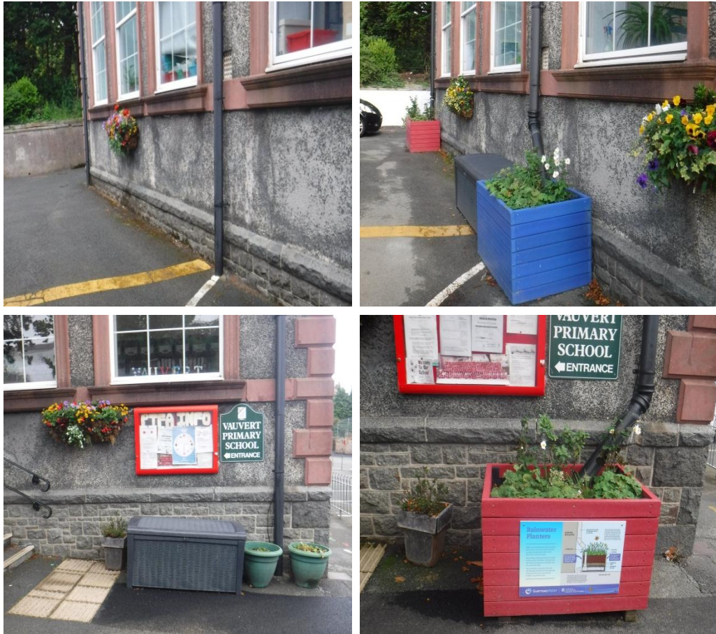
Figure 5: Diverting rainwater pipes through the planters has attenuated surface water from approximately 550m 2 roof areas.
