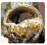
The majority of blockages are caused by cooking fat and oil, which congeal in the sewers, forming a thick layer around the pipe. This prevents sewage from flowing and can cause it to back up. Wet wipes and sanitary items also contribute to some of the worst blockages. Sewer blockages can lead to sewage flooding in people's homes - so please BIN IT, DON'T BLOCK IT!
