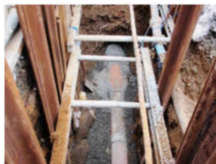
Replaced sewer
