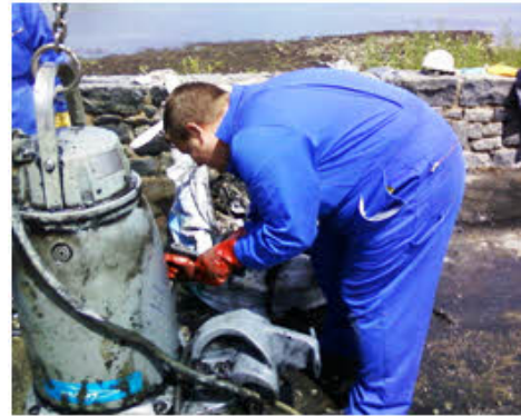
Pump after removal of rags
