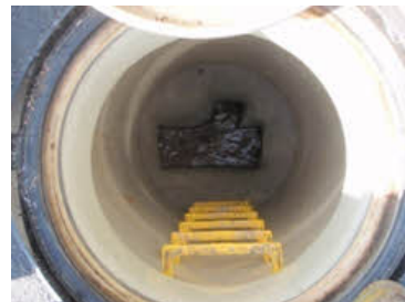
Manhole after refurbishment
