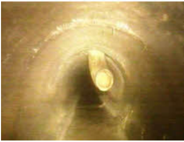
Service intrusion in sewer
