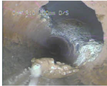
Large hole in sewer
