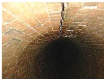
Partial collapse in unlined brick sewer
