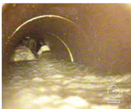
Surcharged sewer before rehabilitation
