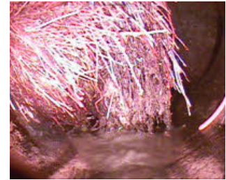
Tree roots protruding into sewer
