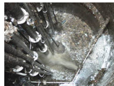
Ingress through penstock at SS Harbour pumping station
