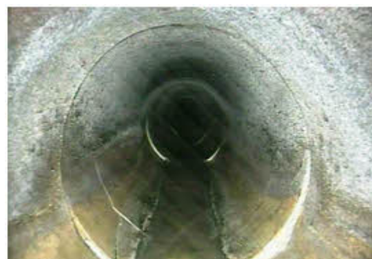
Pipe with multiple fractures
