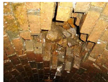
Partial collapse in unlined brick sewer
