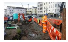
2014 saw the completion of our surface water drainage scheme in Le Truchot (*left*). This provided a surface water sewer to improve drainage, though much more is needed to better understand and manage the risk of flooding in this area. Also in St Peter Port, to minimise disruption the third phase of our Vauvert surface water separation scheme was completed during the school summer holidays.
