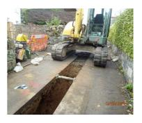
We lined 3.5km of sewer in 2014, following survey work that found them to be in poor condition. In addition, 7 patch repairs were carried out at 4 locations, and 1.3km of pitch fibre sewer in Fort George was renovated. Due to poor condition and high risk of service failure, refurbishment commenced at three of our wastewater pumping stations; Les Goubeys, Les Nicolles and La Mare de Carteret.
