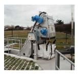
A project finished at the end of the year involved improvements to the raw water pumping capabilities at the Kings Mills station. These works expanded the capabilities of the station by allowing raw water to be moved from one tank to another, and once again involved the installation of a new mechanical screen.
