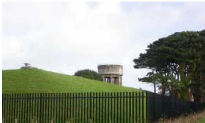
Forest Road Service Reservoirs East, West and Tower
