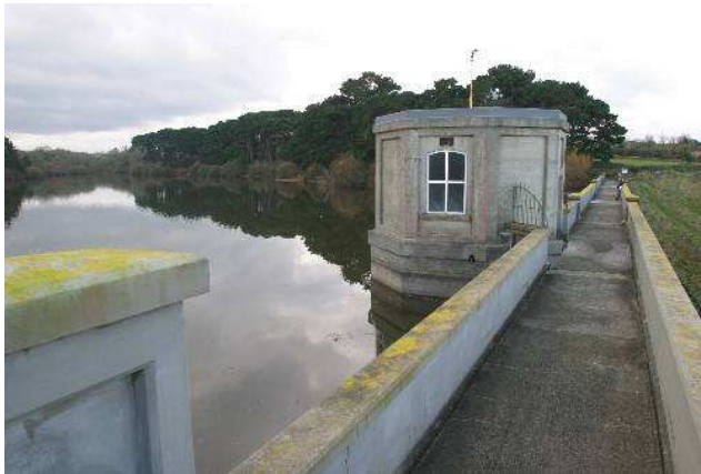
St Saviours reservoir
