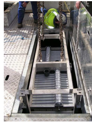
Membrane cassettes being installed
