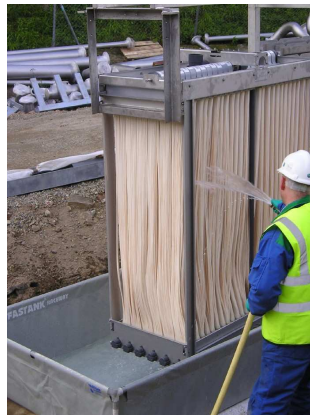
Membrane cassettes being dampened before installation
