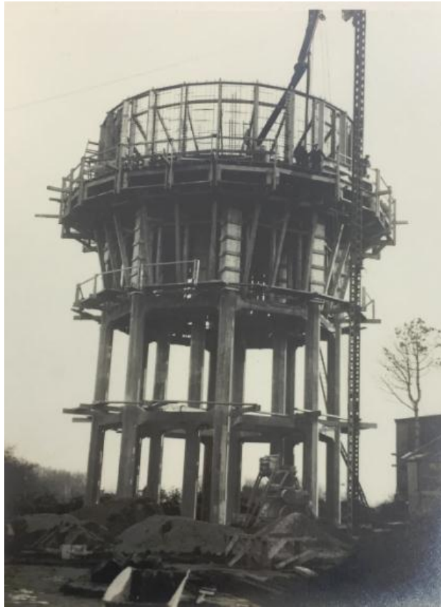
Forest Road Water Tower, built in 1931/32. Constructed to gravity feed properties in the area with treated water in order to balance the peaks and troughs of customer demand.
